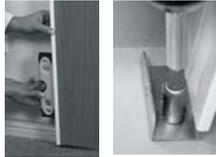
Secure the screw through the bracket and into the bottom of the mounting surface. See the next step if you ordered your shade with a cut-out or you prefer to secure the rail to the side.
