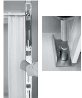
Secure the screw through the bracket and into the mounting surface.
