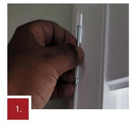
To attach panels, marry the hinges in the frame and panels together. Then drop in the hinge pin to connect. Repeat until all panels are attached. 2.
